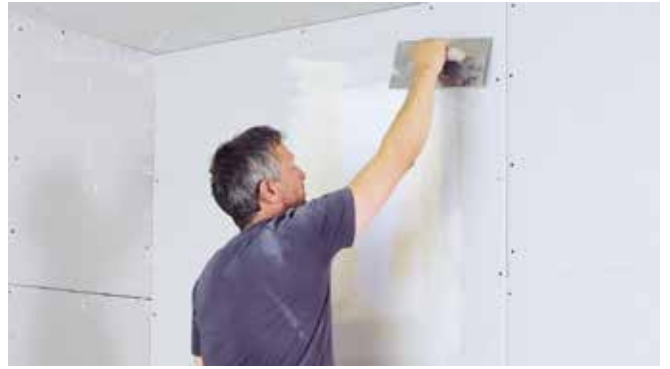
Fill the lining and the surrounding area until a completely smooth surface is created.
