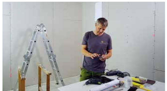
Test the speaker by playing music. The speaker will not produce the correct sound until plastering is complete.
