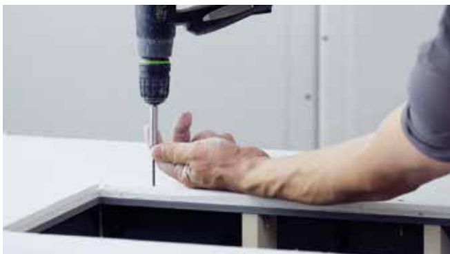
Screw the edge of the back box to the drywall sheet.
