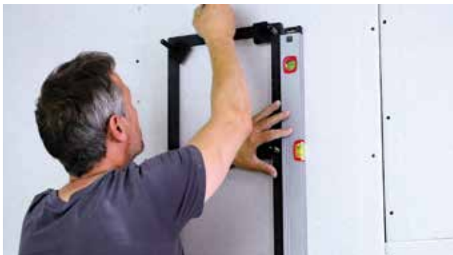
Locate and mark out the installation position. Use the frame as a template (opening).
