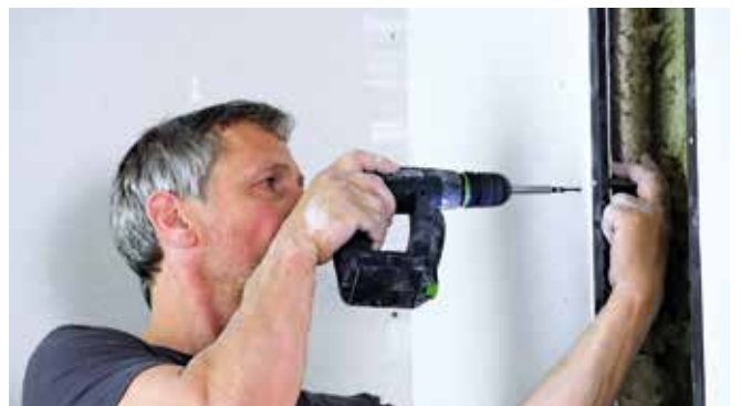
and screw in place.
