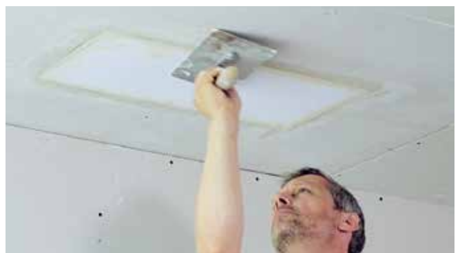
Fill transitions and screw holes without filling the membrane completely.
