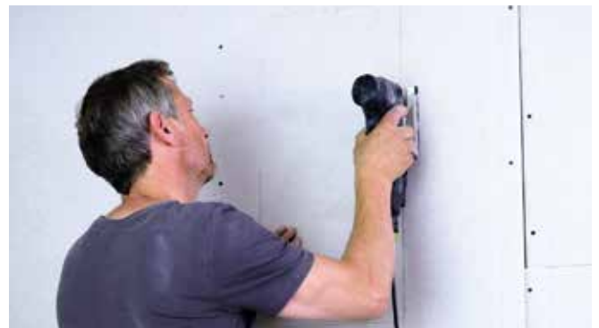
Cut out the opening.
