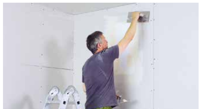
Fill membrane and surrounding area thinly.
