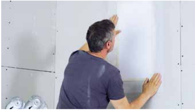
Attach the lining while the plaster is still moist and flatten it. Let it dry and then sand it.
