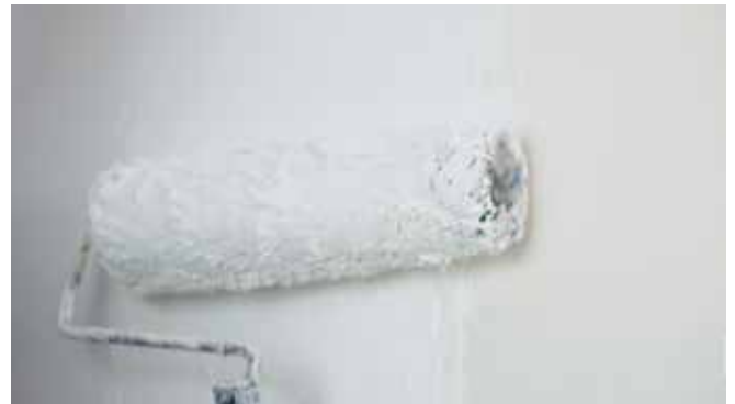
Apply paint. ATTENTION! The plaster must be completely dry!
