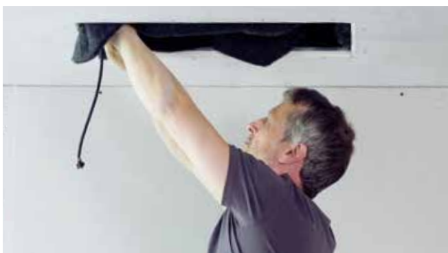
Line the box with the insulating wool...
