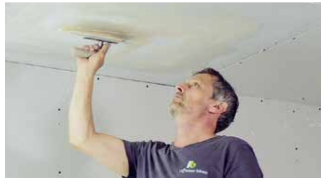
Fill the lining and the surrounding area until a completely smooth surface is created.
