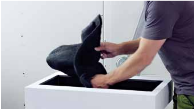
Remove the loose insulating wool from the back box.
