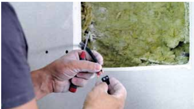
Attach the terminal to the speaker cable. Make sure the polarity is correct.
