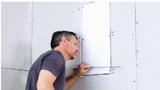
Adjust the speaker so it is flush mounted. The membrane of the loudspeaker must not sit behind the mounting surface but should protrude (max. 1 mm)
