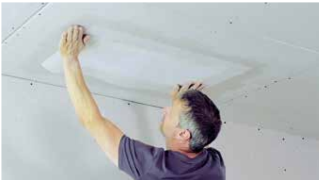
Attach the lining while the plaster is still moist and flatten it. Let it dry and then sand it.
