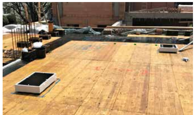
Positioning the back box on the formwork
