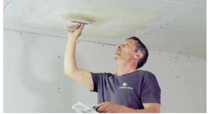
Fill membrane and surrounding area thinly.
