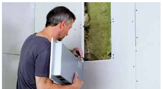
Connect the speaker. Tighten the cable tie.
