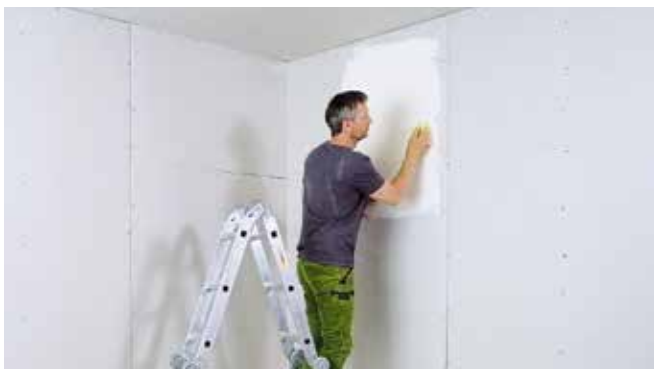
Sand the entire surface. Only apply light pressure over the membrane.
