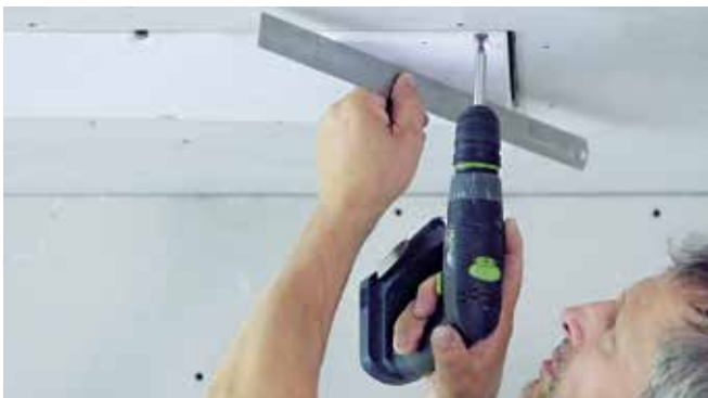
Fix all the screws and adjust the speaker so it is flush mounted. The membrane of the loudspeaker must not sit behind the mounting surface but should protrude (max. 1 mm)
