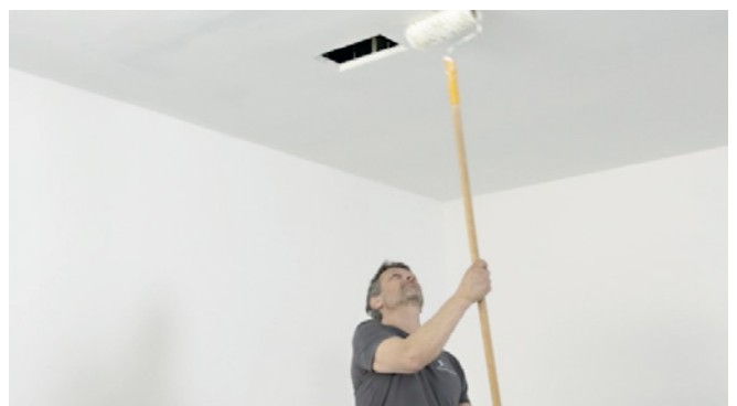
Paint the entire area.
