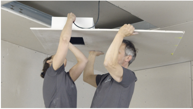
Guide the cable into the back box and seal the cable hole.
