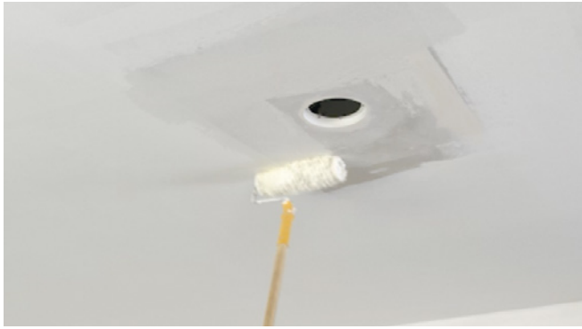
Paint the entire area.
