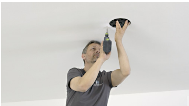
Insert speaker unit and fix in place.
