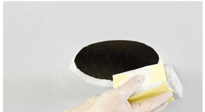
Sand the edges so that no paper residue remains.
