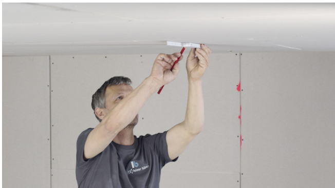
Locate and mark out the installation position.
