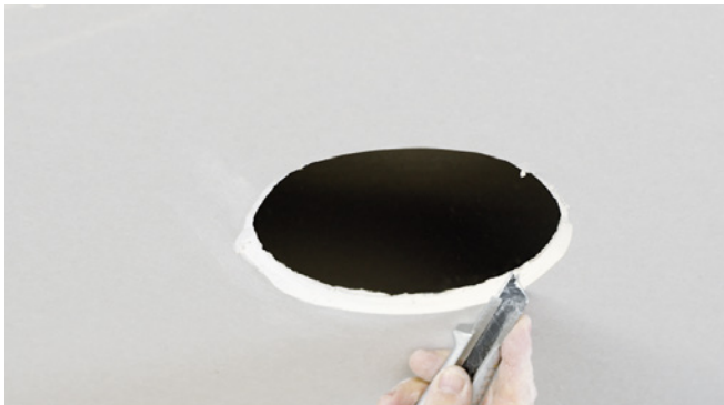
Trim the installation opening.
