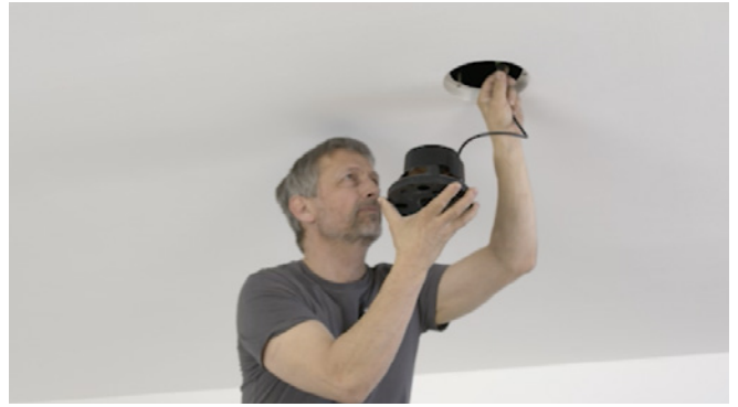
Insert cable of speaker unit into crossover.
