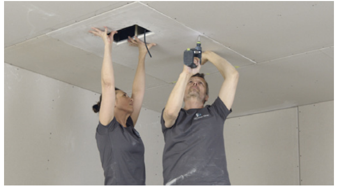
Screw the plasterboard in place.
