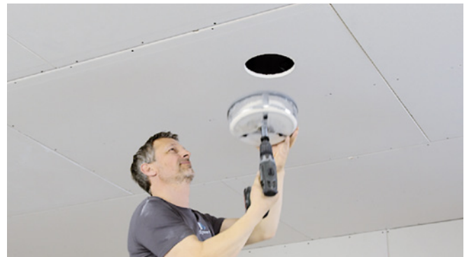
Cut the installation opening. For square openings use a saw to cut out the installation opening.
